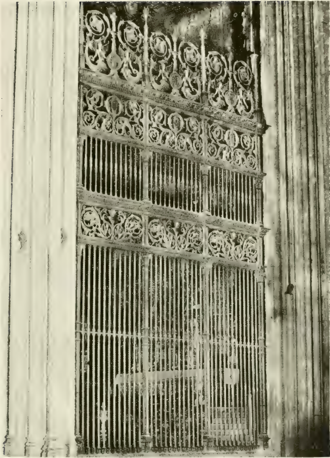
IRON RAILINGS OF THE LATERAL PART OF THE HIGH ALTAR.
